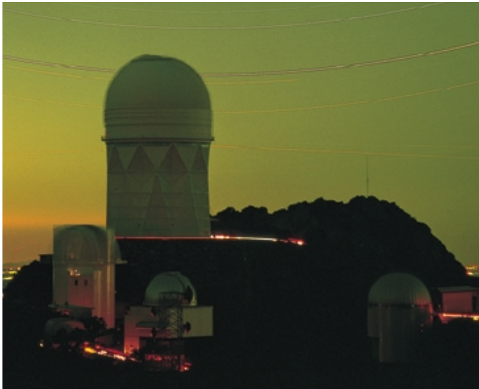
Figure 3.3 This photograph is a time exposure image of star trails over the dome of the Mayall telescope at the Kitt Peak National Observatory in Arizona, USA. The telescope's high-altitude location (over 2000 m) and the clear desert skies reduce atmospheric interference to incoming light.
